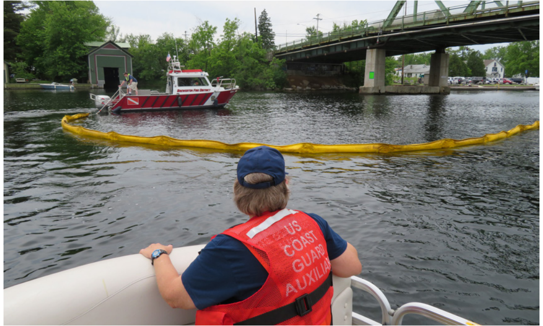
Brewerton Fire Department's marine vessel deploys oil boom in Oneida Lake exercise.
