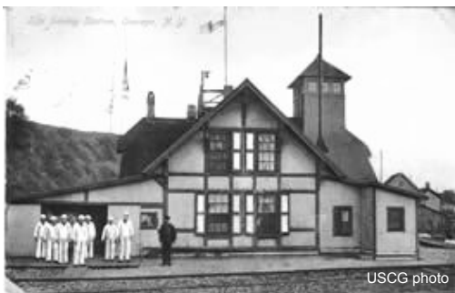
Station Oswego - east side of Oswego River
